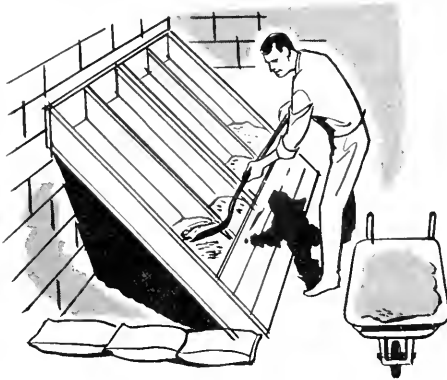
This sand-filled lean-to basement shelter will accommodate three persons. The house itself gives partial shielding. Sandbags are used to block the end of the shelter.
